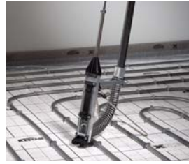
Pipe anchors pre-loaded in magazine.
