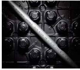
Laid diagonally without tools.
