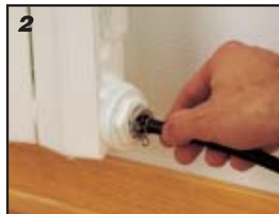
2 Screw on the drain tube provided
